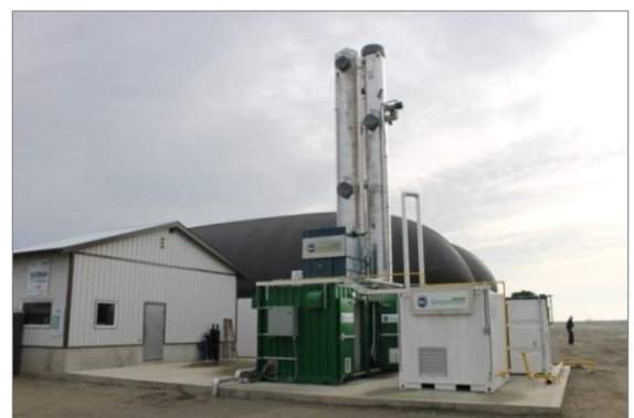
Figure 18. Biogas treatment towers produce RNG, Seebreeze Dairy, Delta, BC (WSU Energy Program)
