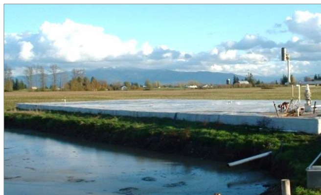
Figure 12. Plug-flow digester at the Vander Haak Dairy (WSU Energy Program)
