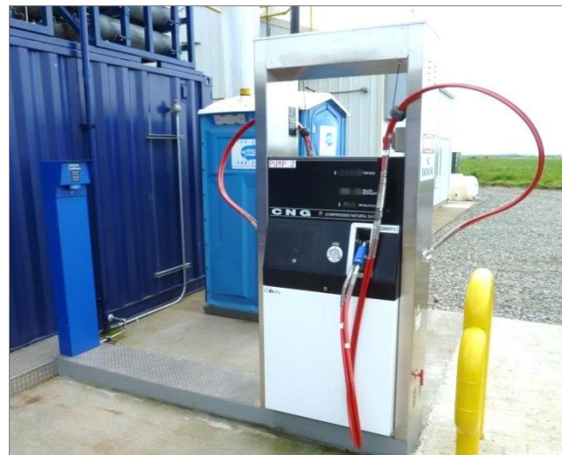
Figure 11. CNG fueling pump (WSU Energy Program)
