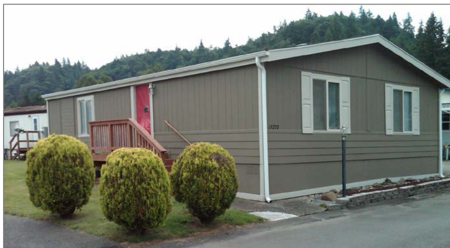
Figure 2. Double Wide Rehabilitated Home at Wonderland
