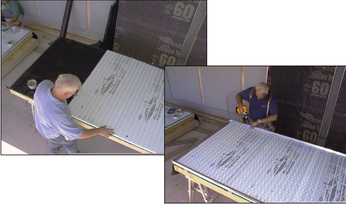
Figure 16 Foam sheathing prior to the application of stucco
