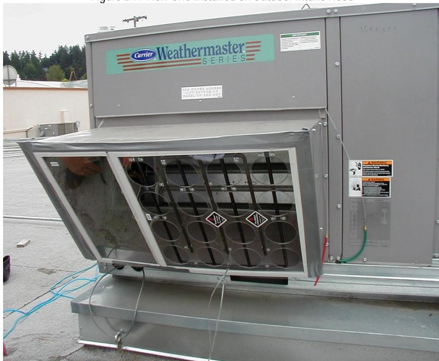
The mixed air temperature is often subject to “plumes” of differing temperature, so at least three measurements of mixed air are taken. Mixed air and outside air temperature can be used as another
