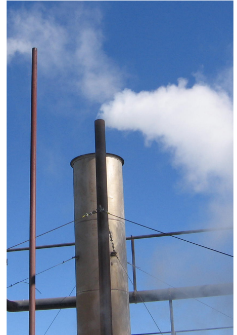
Stack exhaust is a good example of recoverable waste heat in a plant.
