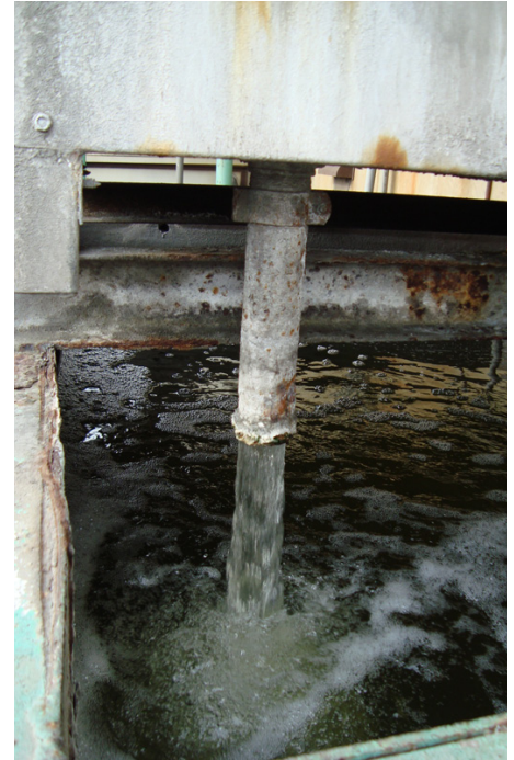
This cooling tower water discharge could be evaluated for possible heat recovery.
