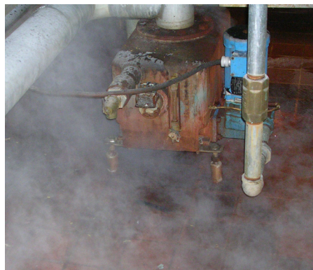
Document the number of steam and condensate leaks while observing steam end uses.
