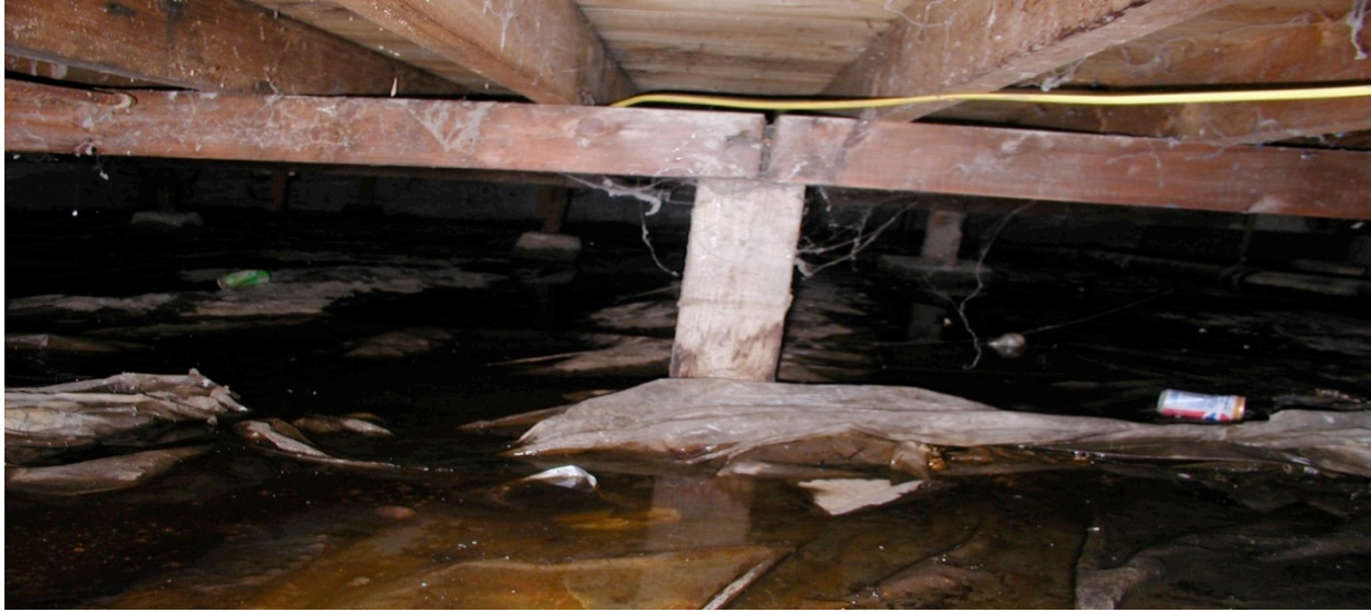
Figure 7. Standing water in a crawlspace: 40 percent of the air you breathe can come from the crawlspace, pulled up by the force of warm air rising. Excess crawlspace moisture is bad for your health, bad for the structure, and a significant factor driving relative humidity UP upstairs.
