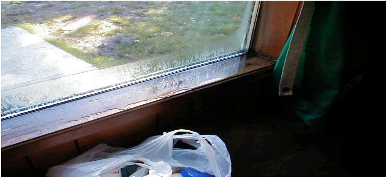
Figure 2. Too much moisture in the air (high relative humidity) leads to unwanted condensation on cool surfaces like double pane windows in cold weather. The moisture drips down, accumulates on sills, and can leak into wall cavities below causing hidden mold growth on wood and paper backed wallboard. Single pane windows will be colder still, resulting in condensation even with normal indoor humidity levels (below 40%) and may require daily drying of sills with towels to prevent mold growth and water damage.
