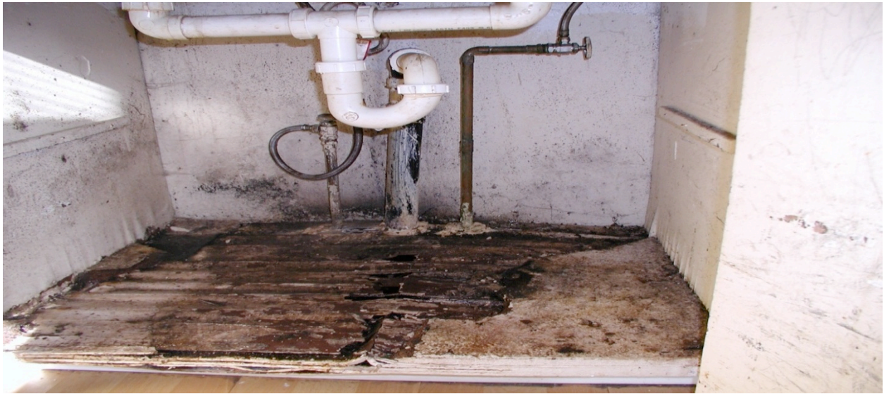
Figure 9. Plumbing leak: Prompt communication with a landlord could have prevented this damage.
