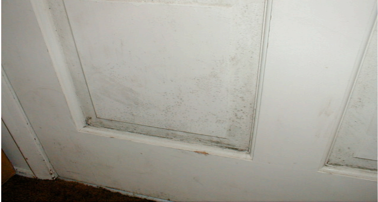
Figure 6. Condensation: Mold growth on inside surface of exterior door. Again, cold surface meets moist air, gets wet and supports mold growth. This can be washed off and repainted.
