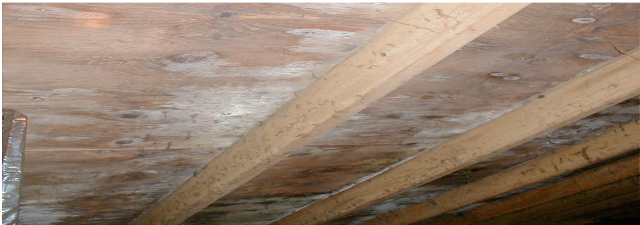
Figure 8. Condensation: Mold growing on roof "sheathing" in an attic. In winter months, moisture (water vapor) leaking through the ceiling of the living area with the force of warm air rising will condense on the cold attic sheathing, causing property damage and mold exposure to occupants. Left uncorrected, the roof will fail and need replacement.
