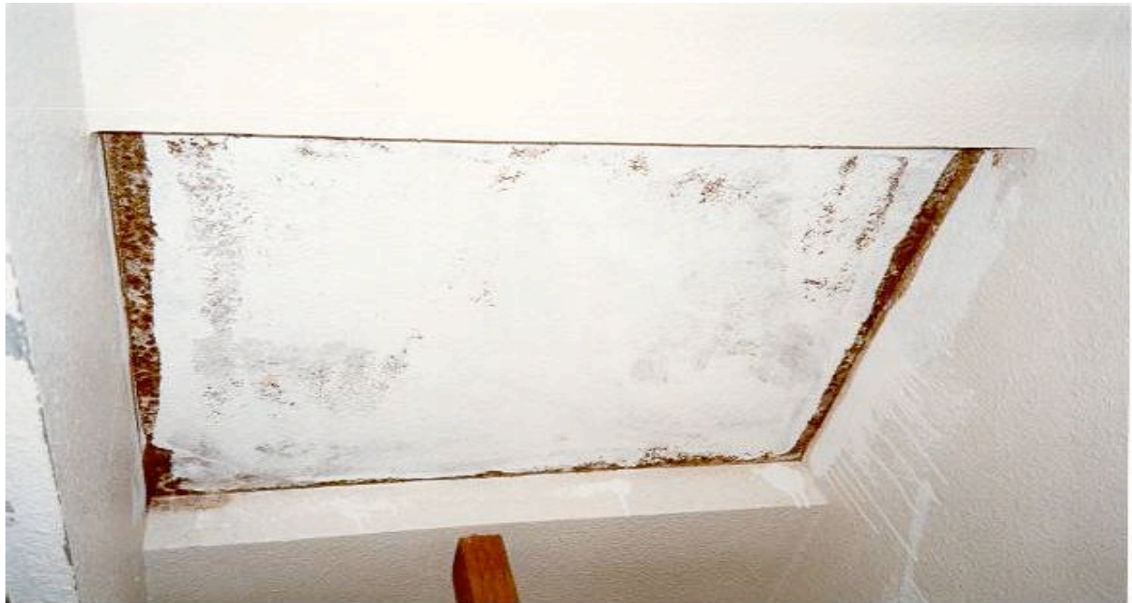
Figure 13. Drywall covered with mold needs to be carefully removed. Painting over mold is not acceptable work practice.
