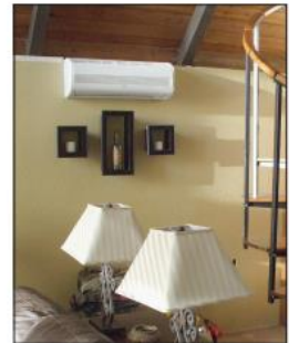
Air handler with blower and heat exchange coil
