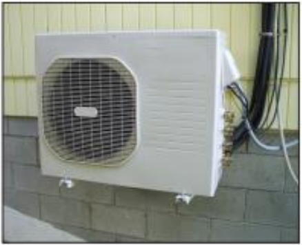
Outdoor unit with compressor and heat exchange coil
