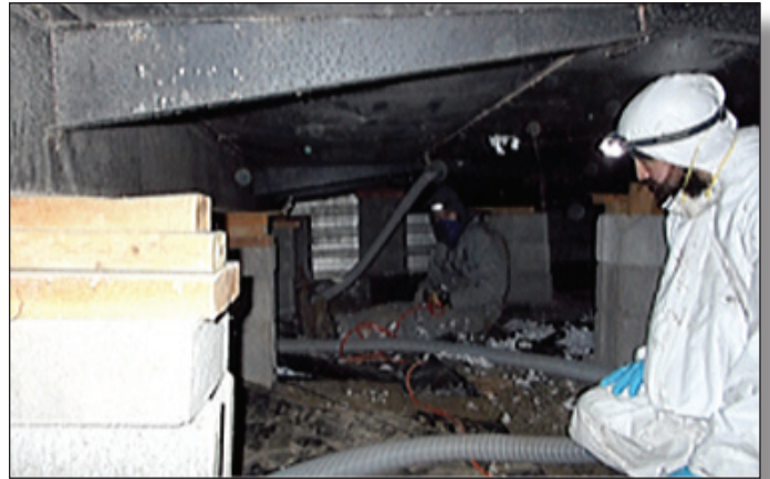
CEEP contractor installing insulation in a residential crawl space.
