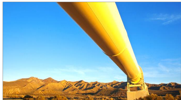
Renewable diesel pipeline
