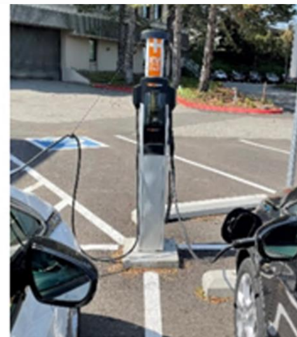
Single pedestal EVSE serving three spaces including an ADA-compliant space. WSDOT, Shoreline (Photo: WSU)
