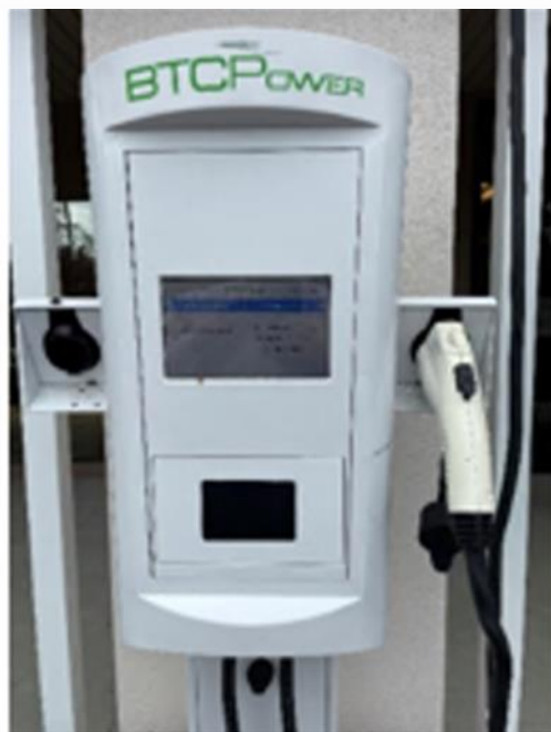
Dual-port wall-mount unit attached to a building column. Shows L2 J1772 plug. Dept. of Commerce, Olympia (Photo: WSU)
