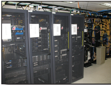
Hot air is expelled from the back of the racked components in the WSU Energy Program data center
